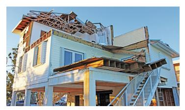
HOME BUILT UNDER OUTDATED BUILDING CODES AND STANDARDS Roof structure loss and collapse of the second-floor exterior wall and adjacent deck incurred after Hurricane Irma by a pre-FBC home.
