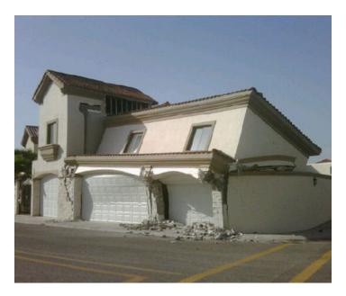
SOFT STORY COLLAPSE DURING THE 2010 MEXICALI EASTER EARTHQUAKE Soft story buildings consist of large, unreinforced openings on their ground floors and are susceptible to failure during an earthquake due to their inability to withstand large lateral forces. When the first floor collapses, the upper levels are no longer supported and will also collapse.
