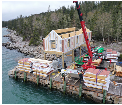
Highly insulated, floodplain-elevated, demountable biogenic assembly for completely off-grid remote wet laboratory.
